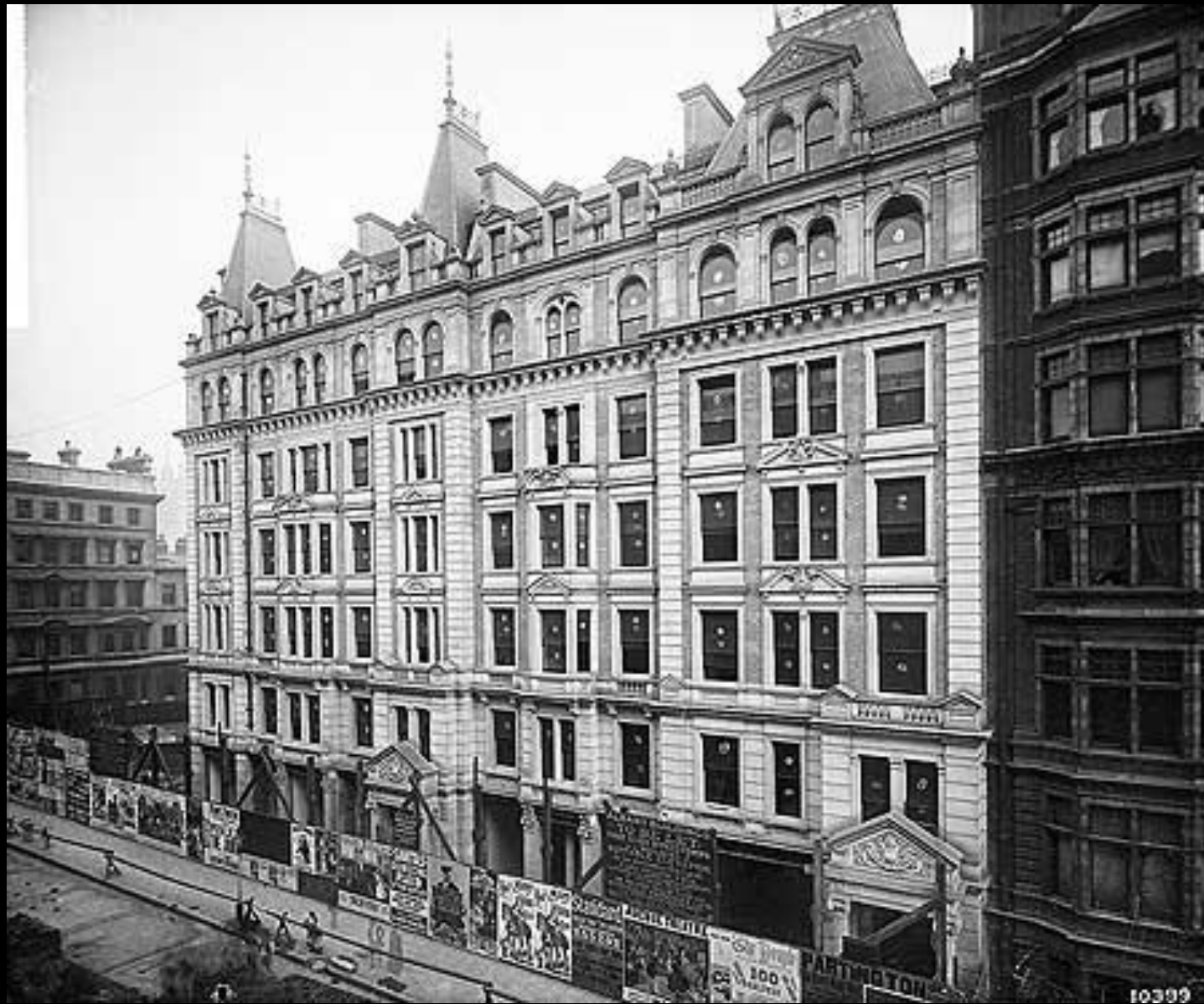
Albany Buildings, 47 Victoria Street, Westminster, London. Historic England BL10399
